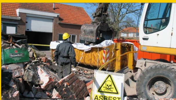
Asbestsanering Sint Laurens.
