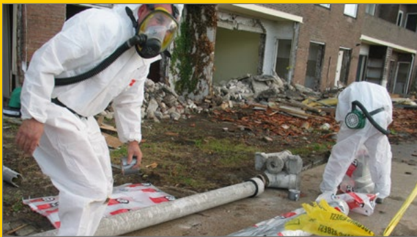
Sanering asbest cement leiding.
